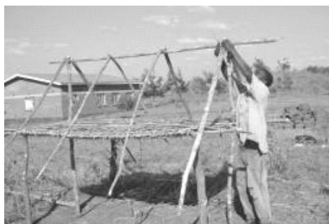
Step 1: Making the structure, similar to a local Tandala in Malawi
